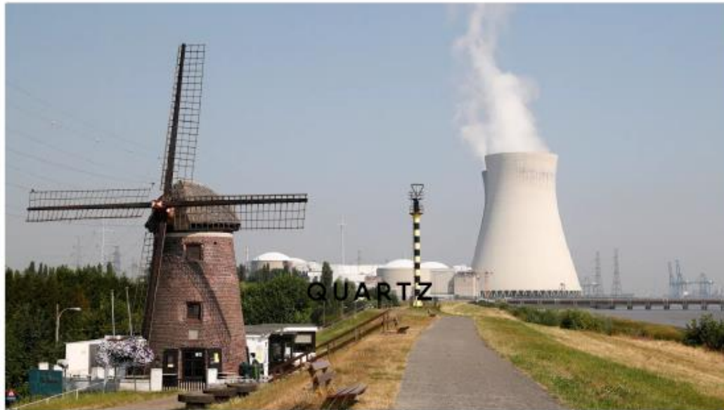
Towers of power.
