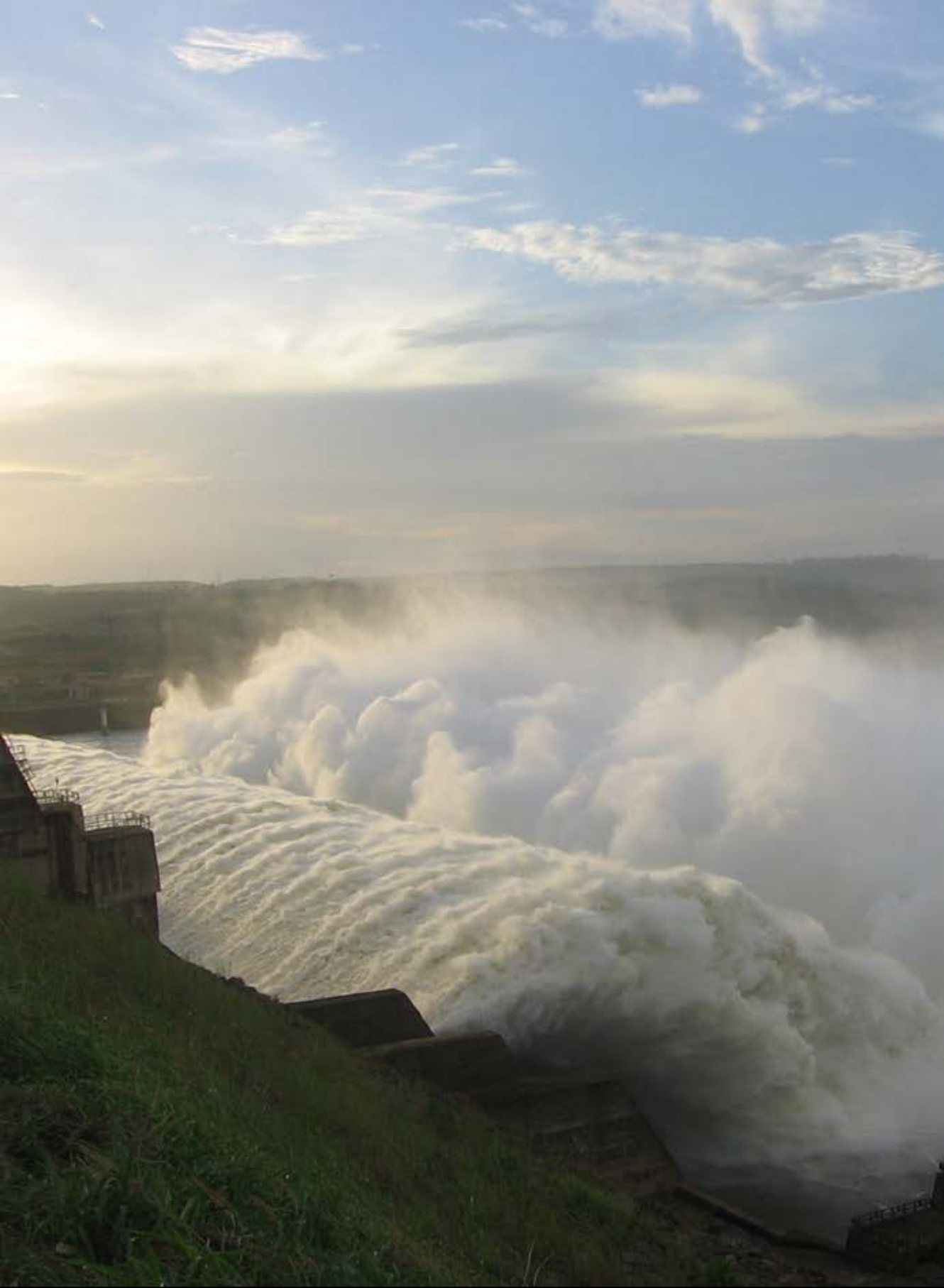
Tucuruí Dam spillway, Tocantins River, Brazil. Photo: © Eneida Castro
